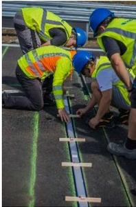
It only takes a few hours to install Weigh In Motion technology: a narrow strip is sawn out of the asphalt to accommodate the sensor technology.
