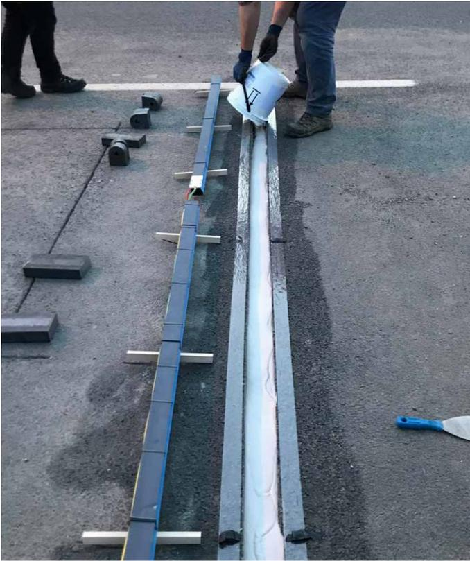
Before the Kistler Linesas WIM sensor is installed, the slot has to be filled with a grouting compound. This is a 3-component epoxy resin composition, specially developed for this installation.
