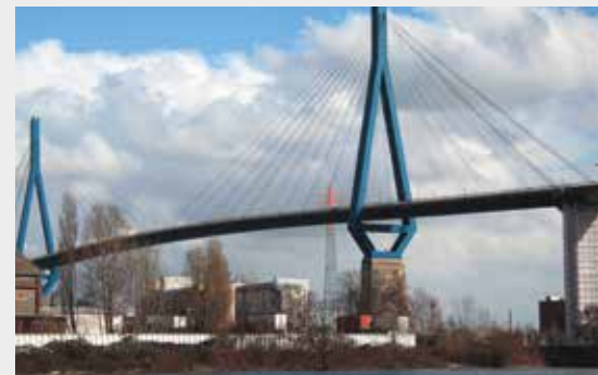
Koehlbrand Bridge in Hamburg, Germany
