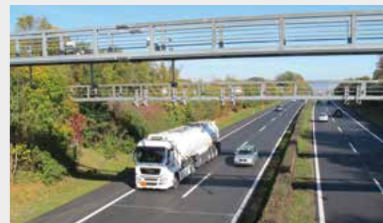
Free flow toll collection system in Switzerland
