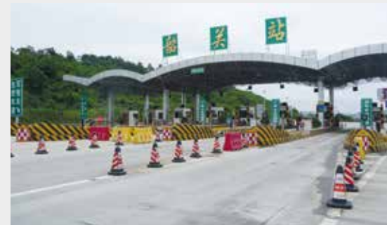
Toll plaza with Lineas® WIM sensors in China
