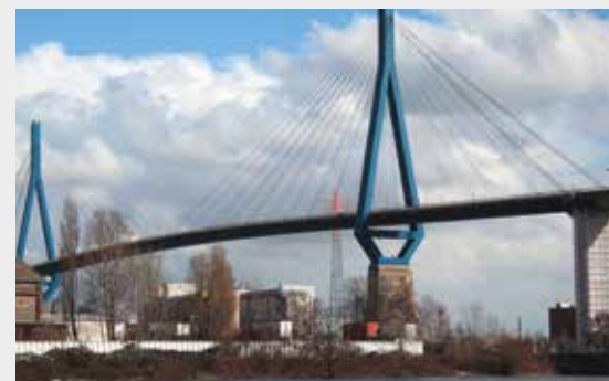
Koehlbrand Bridge in Hamburg, Germany
