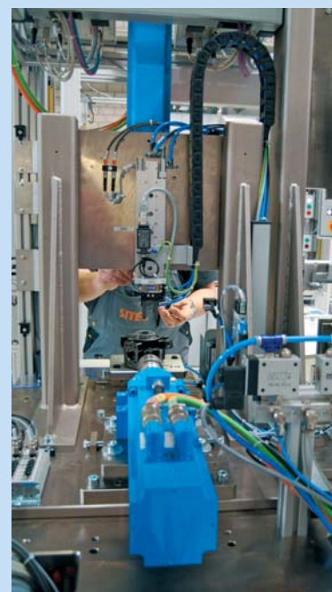
Assembly with NC servo presses in factory of special machinery manufacturer SITEC
